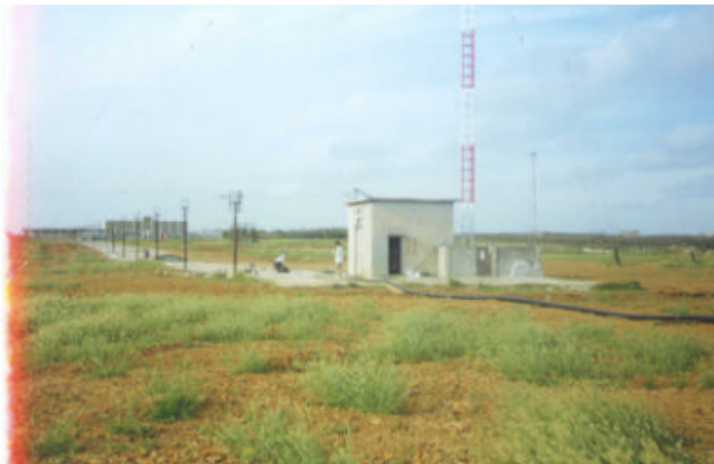
Fig. 1 The AM \lambda/4 dipole antenna tower, 66m in height, operating at 1143 kHz, located in Peihou, Taiwan, and owned by Taiwan Fishery Station
